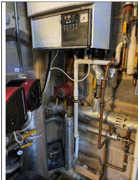
Figure 27: Unlagged pipework
