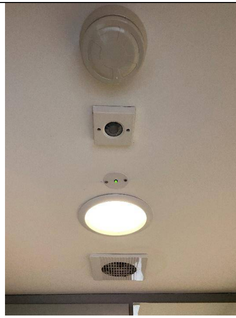
Figure 26: PIR movement controls in toilets
