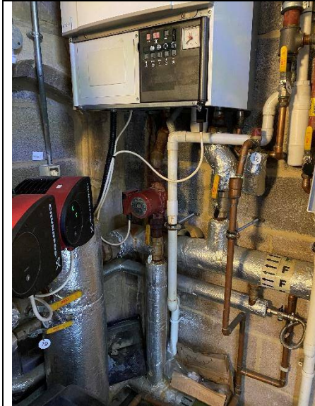
Figure 10: Unlagged pipework
