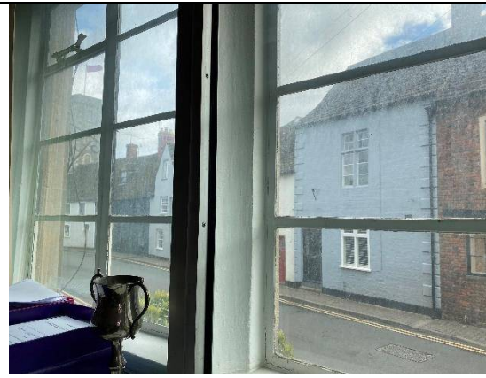
Figure 20: Example of retrofit double-glazed interior windows to reduce heat loss
