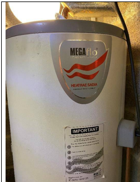
Figure 15: MegaFlo CL250HE electric immersion heater
