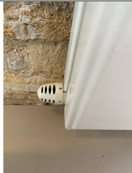
Figure 13: Thermostatic radiator valve
