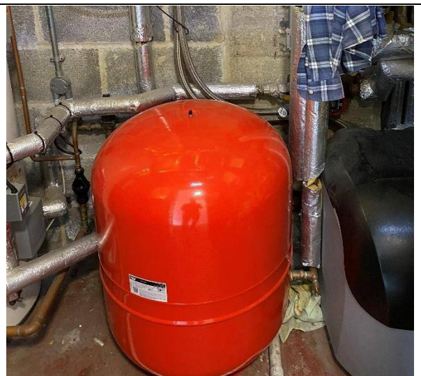
Figure 16: Zilmet expansion tank
