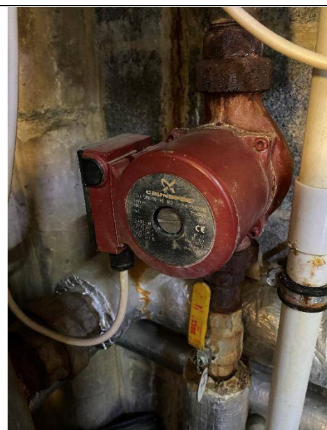
Figure 9: Unlagged Pumps
