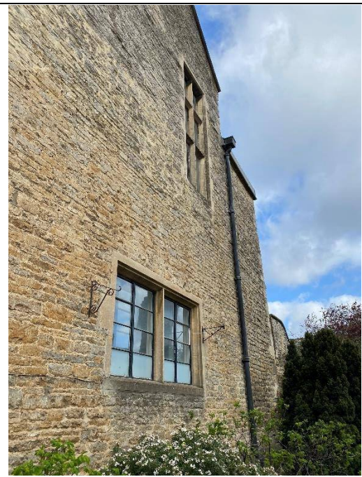
Figure 4: External shot looking at the building from the west side
